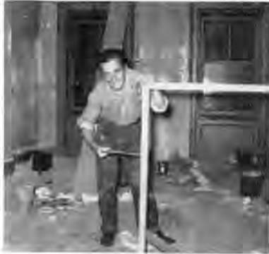
Joe Cicio doing his part renovating the New Eta House.
